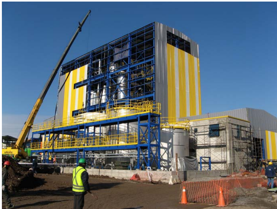
Fig. 5: Industrial plant in the late erection phase
