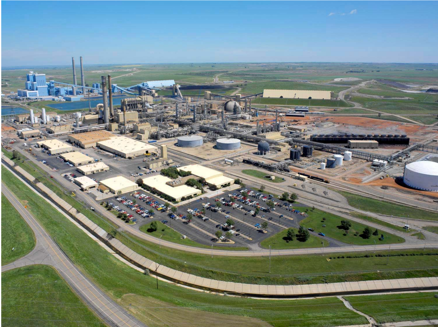
Figure 9 Basin Electric's Antelope Valley Station (in background) and Dakota Gasification Company's Facility (in foreground)
