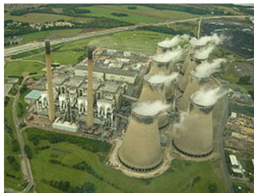
Figure 7 Ferrybridge power station
