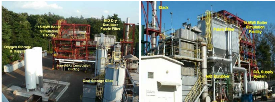
Figure 5: BSF after oxy-firing modifications
