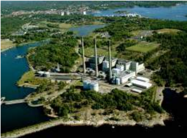
Karlshamn Power Plant (Sweden)
