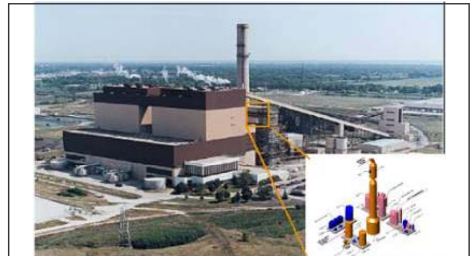
5 MW Pilot Plant (USA)
