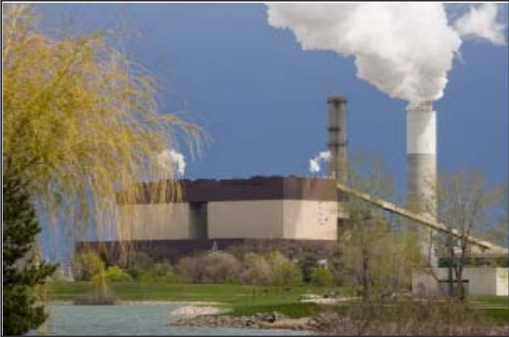
Pleasant Prairie Power Plant (US)
