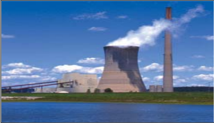
Industrial demonstrator 30 MWt, Mountaineer (US)
