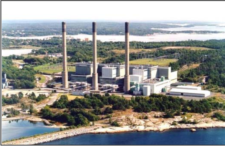
Karlshamn Power Plant (Sweden)
