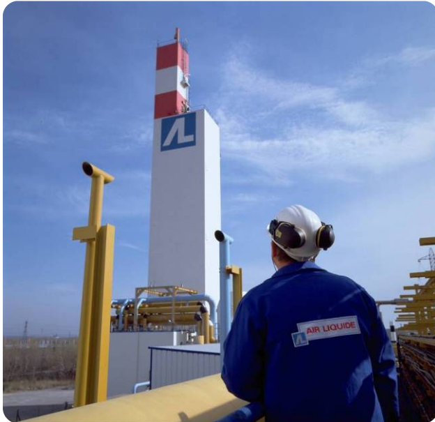
Air Separation Unit (ASU)
