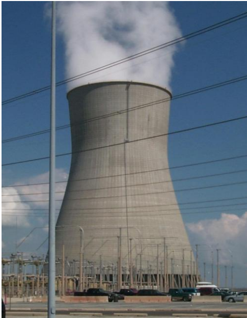
Cooling Tower $ 400m.....
