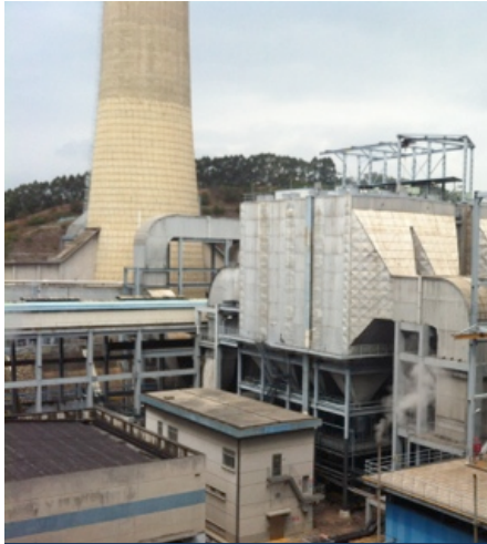
Shajiao Power Plant, Shenzhen
