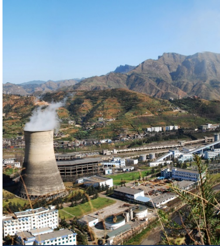
Yixing Power, Jiangsu
