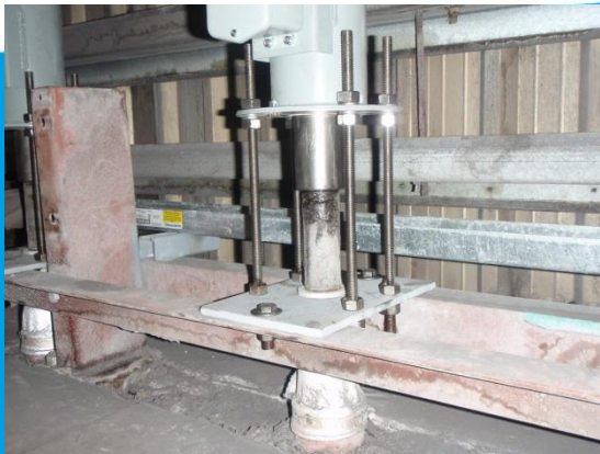
Tumbling Hammer to Magnetic Rapper Conversion
