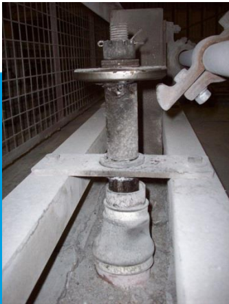
Tumbling Hammer to Magnetic Rapper Conversion
