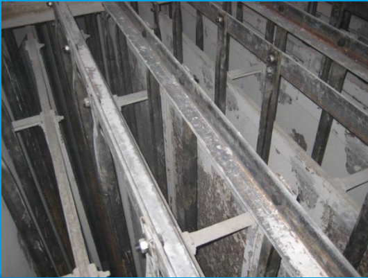
New Rigid Electrode System
