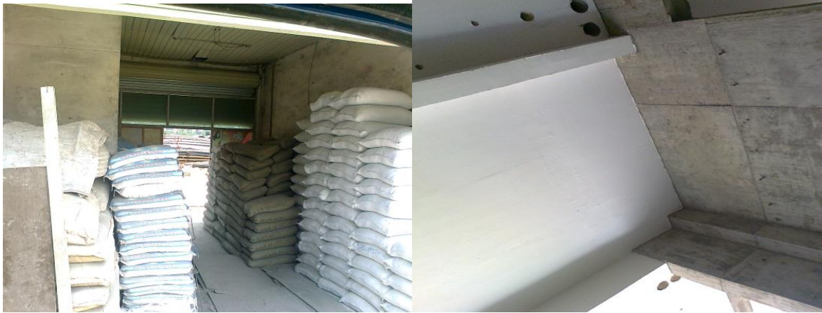
Figure 10 Mortar Application with Dry FGD By-Product (bagged) Addition
