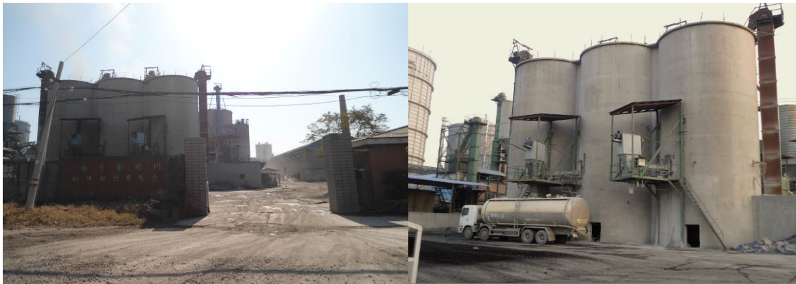
Figure 9 Operation Plant of GGBS Production with Dry FGD By-Product Addition
