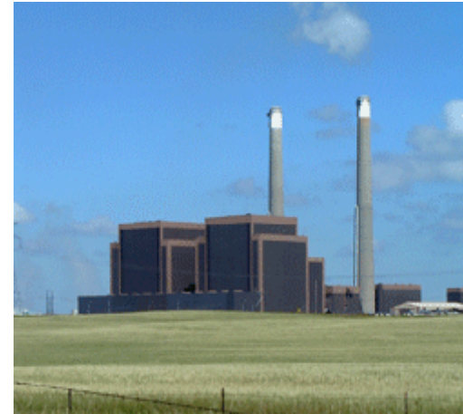
Great River Energy Coal Creek Station
