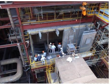
Since the SCR required a minimal volume of catalyst, the necessary duct changes were greatly reduced. This allowed most of the existing duct work to be used in the new design and allowed for 1 week tie-in outage installation.
