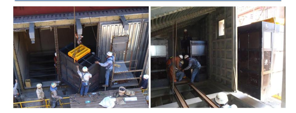
Because the design minimized the necessary catalyst volume, the catalyst install could be completed in two working days.
