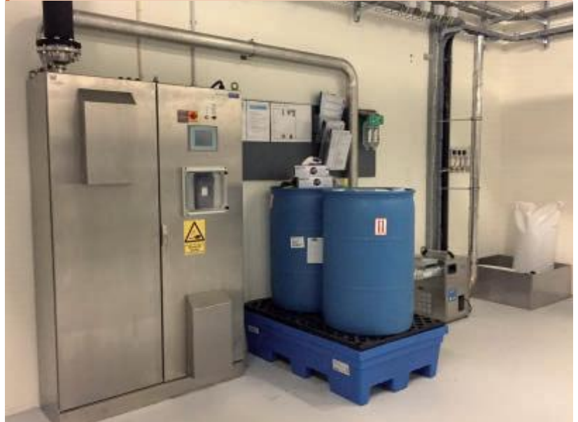
Figure 4: VPHP integrated generator with a continuous desiccant and bulk source or hydrogen peroxide solution
